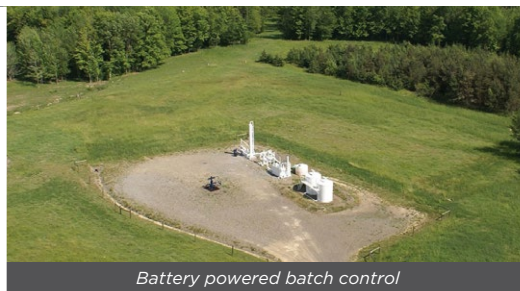
Battery powered batch control
